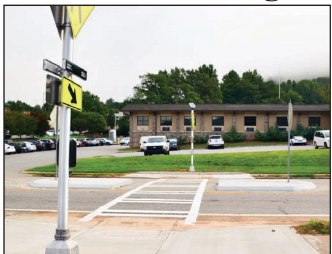
The new GDOT crosswalk at Chatuge Regional Hospital on Main Street was completed Wednesday, July 8. Photo by Lowell Nicholson
